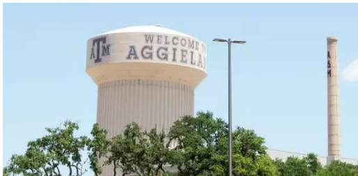
Figure 2 - A&M Water Tower
