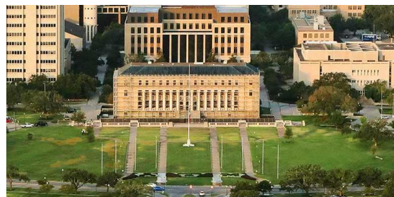
Figure 1 - Jack K. Williams Building
