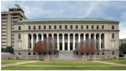
Figure 2 - Texas A&M University, Jack K. Williams Building.
